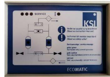
If a dewpoint controller (shown on the right here) is used, then the operating status is also shown. Arrow keys can be used to display much information about the current status.
